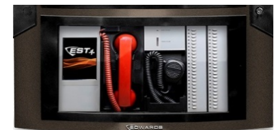
Public Address and Evacuation Audio, Telephone Firefighter Console
